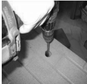
Drilling a Hole for the Gas Line
