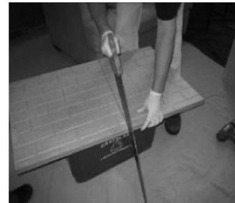
Cutting the Panel to Size
