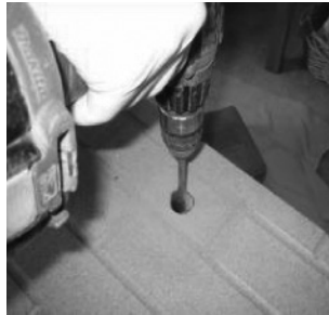
Drilling a Hole for the Gas Line
